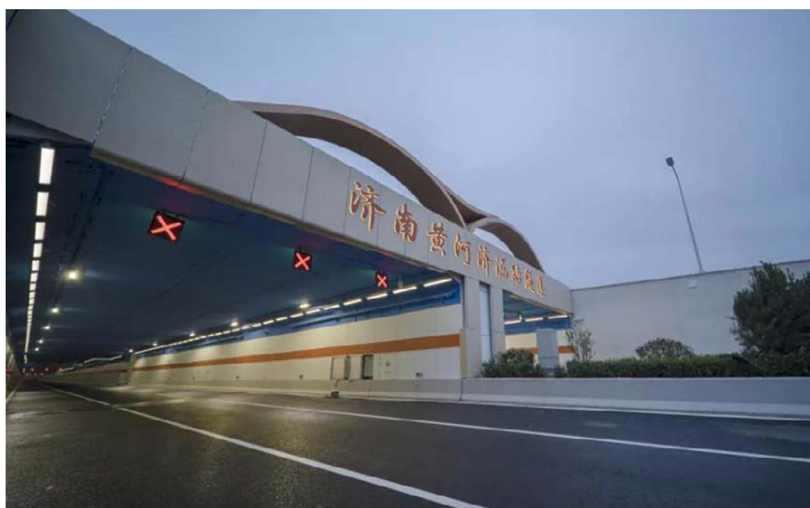
The construction site of Ji'nan tunnel project supported by Shandong Branch.
