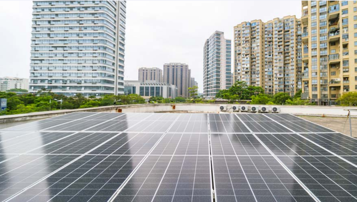
Xiamen Government Affairs Centre Sub-branch installed photovoltaic equipment on the roof to generate electricity.
